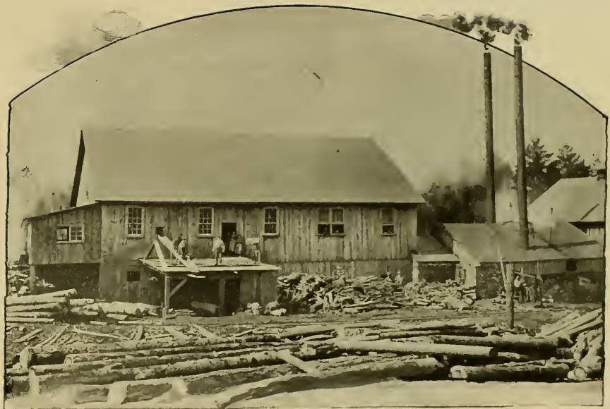
STAUFFER'S MILL, NEAR LAUREL INN, ISAAC STAUFFER, PROP'R.
